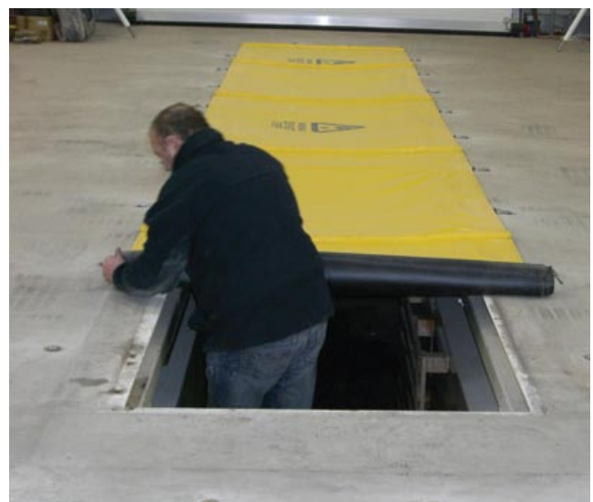
Figure 61 Reinforced fabric cover being fixed in place (photograph courtesy of Everquip Garage Equipment Ltd)
